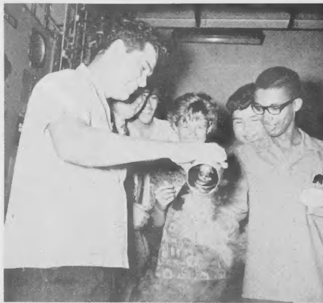
LANG GERMAN demonstrates how liquid nitrogen hardens rubber tube.
